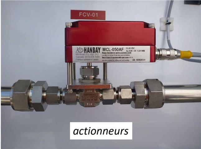
Electric valve **actuator** controlling a ½ needle valve
